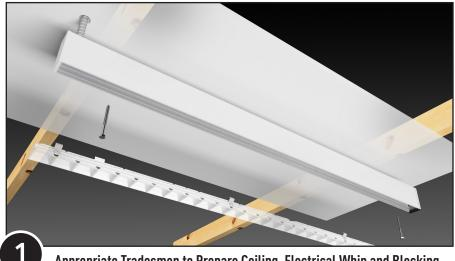
Appropriate Tradesmen to Prepare Ceiling, Electrical Whip and Blocking (or All-Thread) As Shown, and then Make Ceiling Cut-Out
