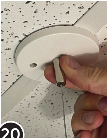
Manually Attach Power Cord and Non-Power Canopies with Suspension Cable Assemblies
