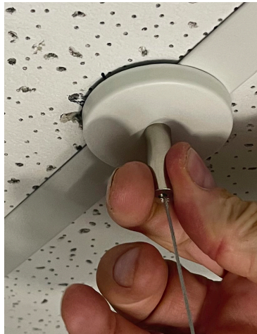
Manually Attach Power Cord and Non-Power Canopies with Suspension Cable Assemblies
