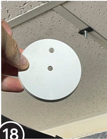
Locate Power Cord Canopy and Prep Ceiling Tile
