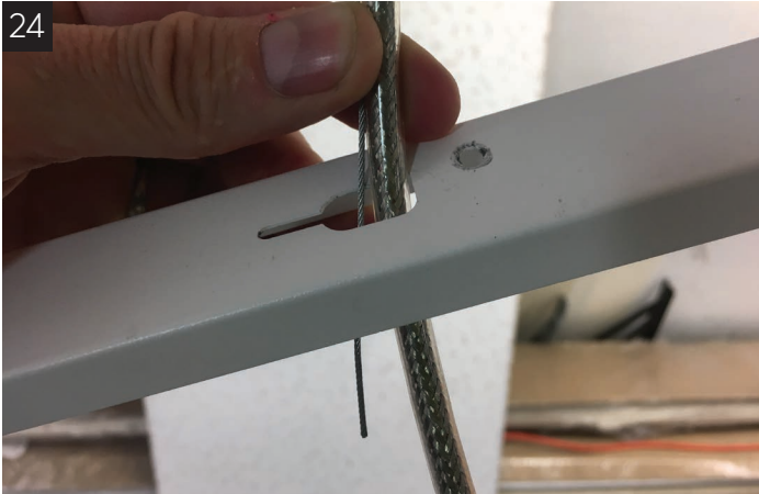
Thread aircraft cable through cover.
