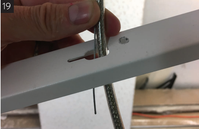
Thread aircraft cable through cover.
